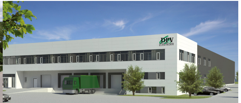
2018 – New building site 2, logistics center Tiefental
