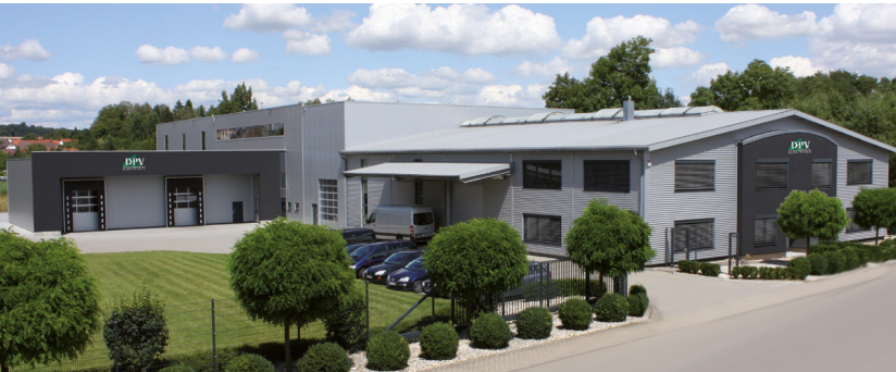
2008 – Triplication of the plant area
